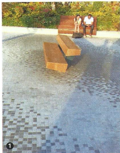
Precedent 1: Pixellation and transition of 2 types of granite colors to create overall pattern
