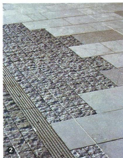
Precedent 2: Interface of 2 types of paving size/ colors and finishing to create transition pattern
